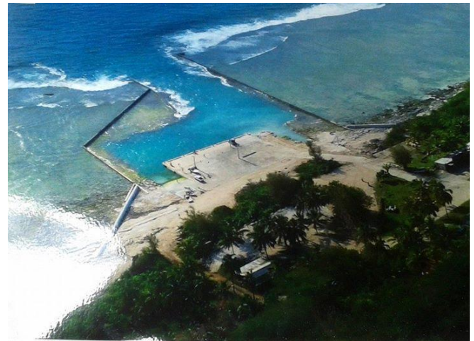
The recently renovated Mangaia Harbour designed by applying the coastal calculator method.
