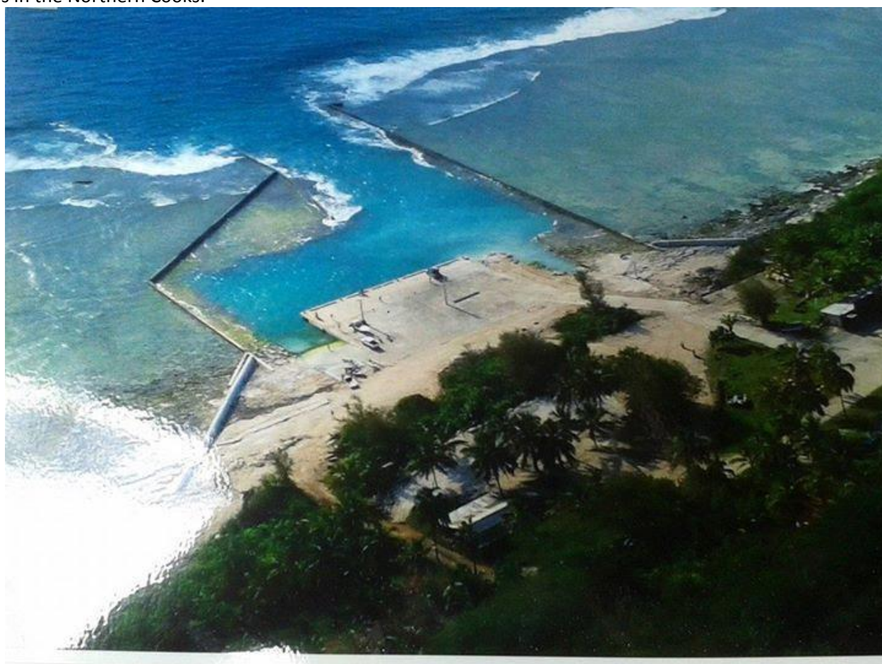
The completed Mangaia harbour 2014 (Picture provided by Paul Maoate ICI)
