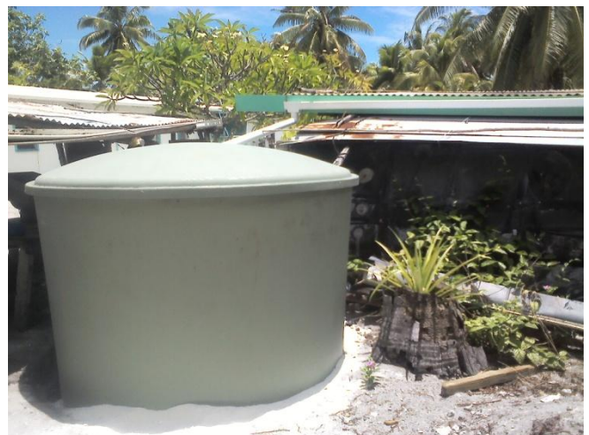
A completed household water tank on Palmerston Island (Photo provided by Arthur Neale)
