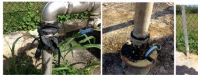
Figure 6 L: Leaky joint inadequately repaired at Mokoero station. C: Moss growth at the b... R: Moss growth at the piping joint at MUK-4A.
