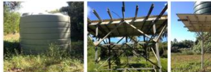
Figure 16 L: The Angiagi tank had no stand. C: The Tinokura station did not ha... R: The Vaimutu tank did not have a proper outlet attached to it.
