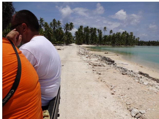
Causeway on Pukapuka knocked about by many cyclones with the final blow from cyclone Ula, reducing it to rubble Feb 2016 (Photo by Celine Dyer)
