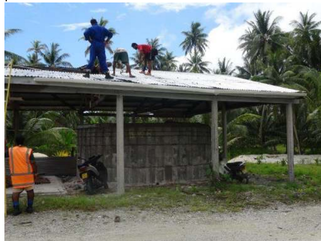
Workmen stripping off the old roof, Photos provided by Lucky Topetai
