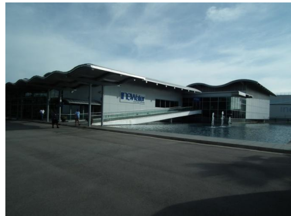
NeWater, one of 4 facilities, that converts waste water into drinking water (Picture by Robert Matapo)
